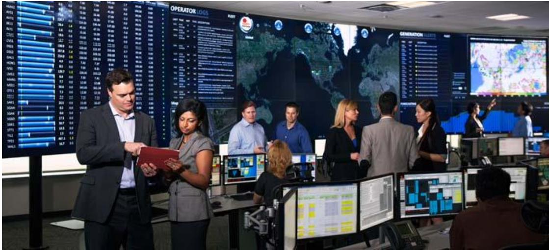
Figure 10. First Solar operations center in Tempe, AZ. Image from First Solar
