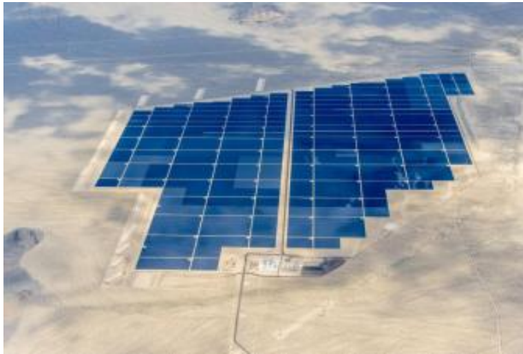
Figure 6. Aerial photo of 300 MW PV power plant (source: First Solar)
